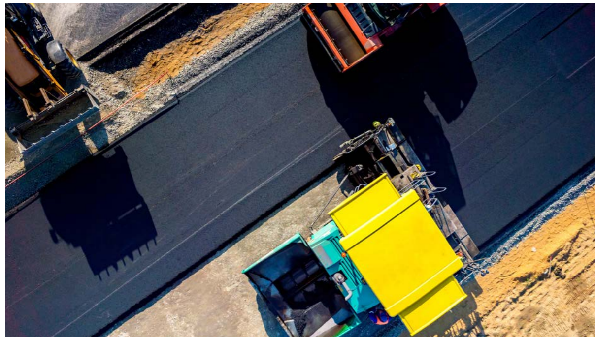
Production of asphalt products using waste oil and sludge from storage tanks
